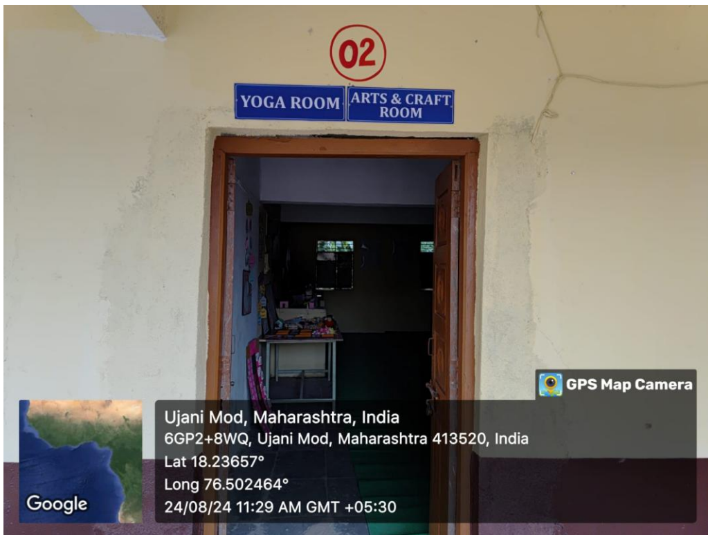
External view of Yoga/Arts & Craft Room (Hall No.02)
