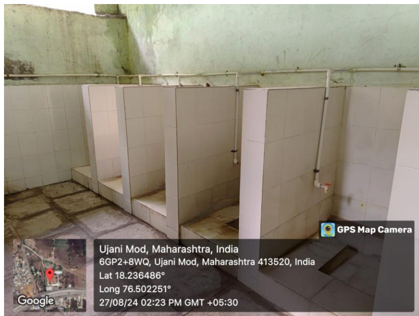
Internal view of Boys Urinal
