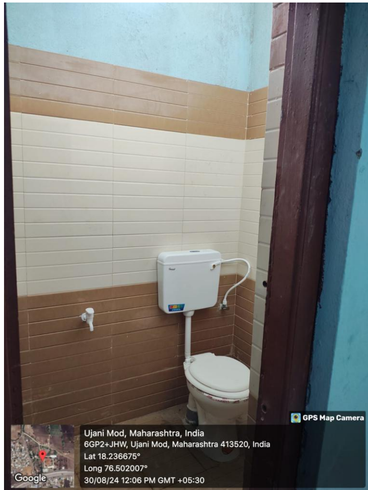
Internal view of Girls Toilet
