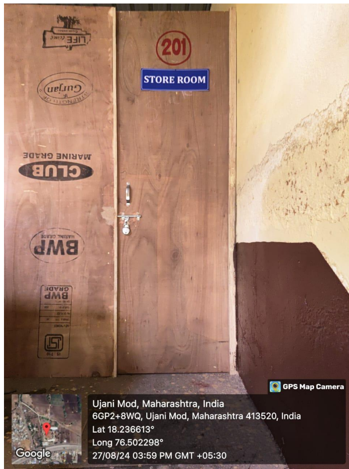
External view of Store Room-(Room No-201)
