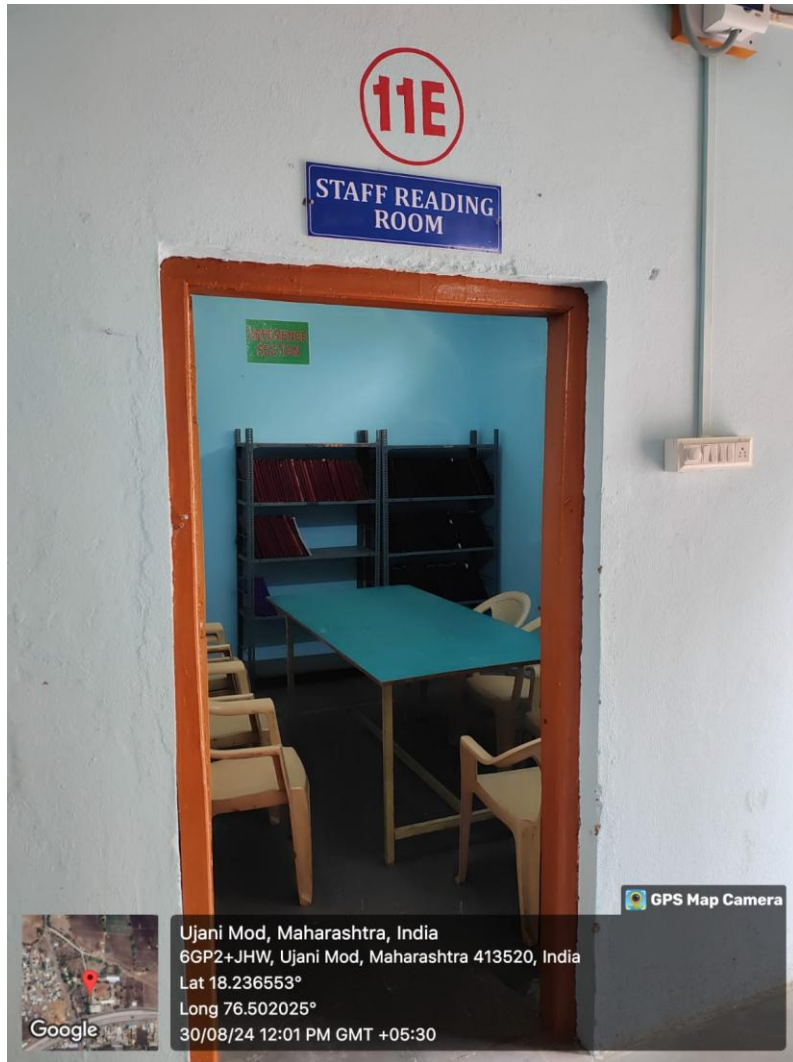
External view of Staff Reading Room (Hall No.11E)
