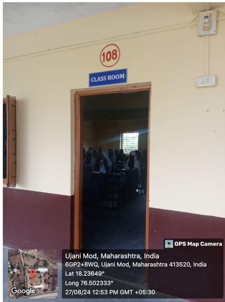
External view of ICT Enabled Classroom-3 (Hall No.108)
